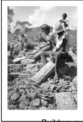
Builders cutting and shaping the stones for the Church.
